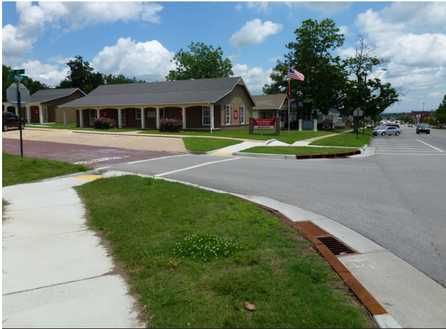
Main Street in Collinsville was retrofitted recently with new ADA-compliant curb cuts, storm drainage and sidewalks.
